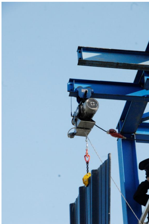
Construction site: Lifting loads with wireless remote control
